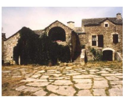
Figure 1: House, Built of stone laid in mud mortar with paving stone yard of stones in mud mortar. Photo: CRATerre/EAG.
